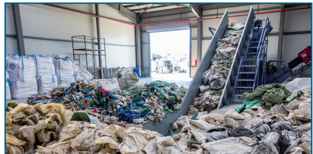
Fig. 2: Underfloor belt conveyors for feeding loose and separated materials
